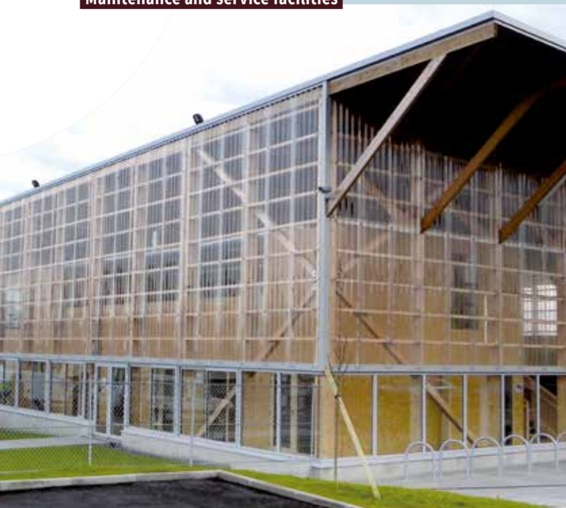
Maintenance and service facilities
